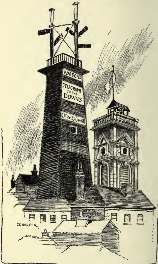
OLD TELEGRAPH TOWER, TOOLEY STREET.
